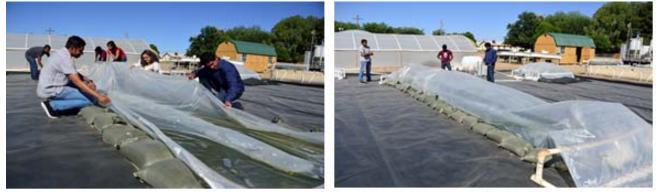
Figure 3. Fabrication of the enclosed photobioreactor for cultivating Galdieria sulphuraria in the POWER process.
