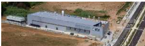
Figure 6 External view of the ST-4 energy plant
