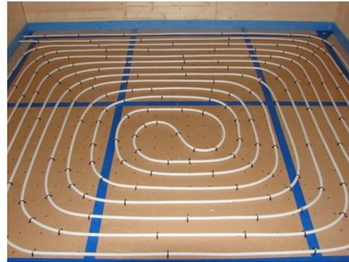
Fig. 7. The floor heating circuit
