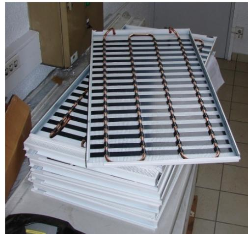
Fig. 8. The chilled ceiling plates
