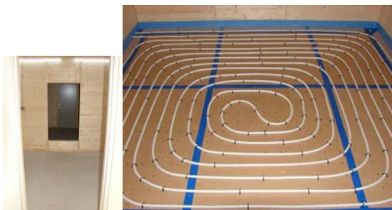
Fig. 9: The hot chamber : (a) Inside the room, (b) Floor heating (before cement screed)
